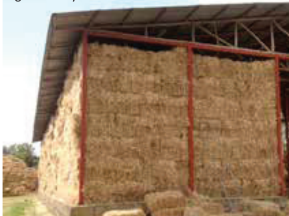
High roof hay store
