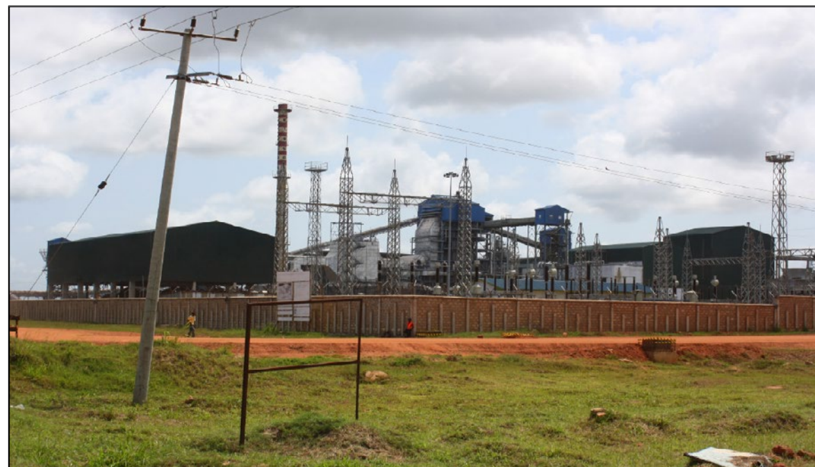
Figure 13: Guarded KISCOL factory area in Kwale
